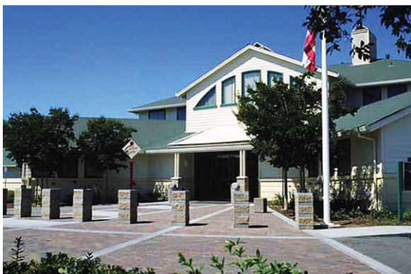
Santa Clara County Children's Shelter
